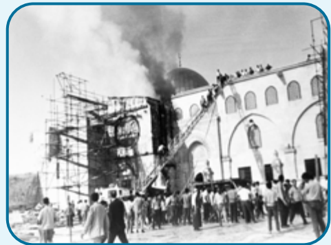
Al-Aqsa Mosque arson 1969
