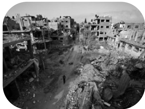
• Buildings destroyed by Israeli shelling in Gaza during the Battle of Sword of Jerusalem
