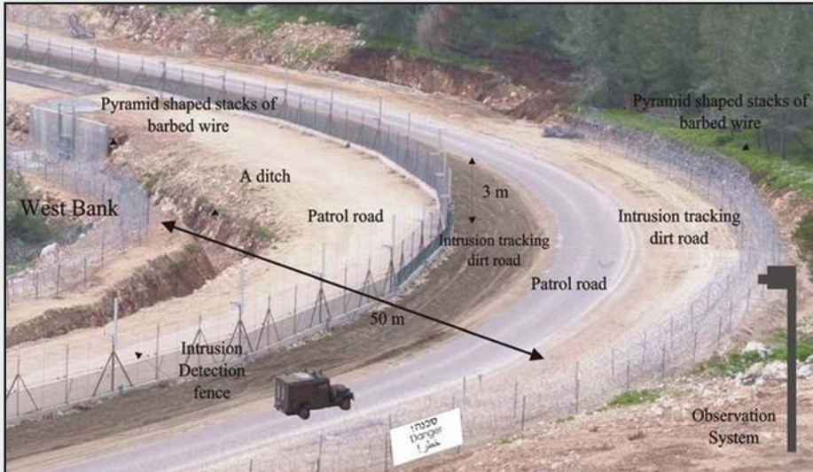
Figure 1: A Section Showing the Structure of the Separation Wall
